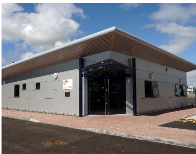
DSA Test Centre (photo: DSA crown copyright)
